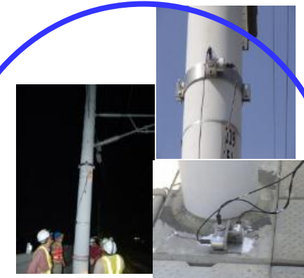
Verify the resonance of viaduct and pole
